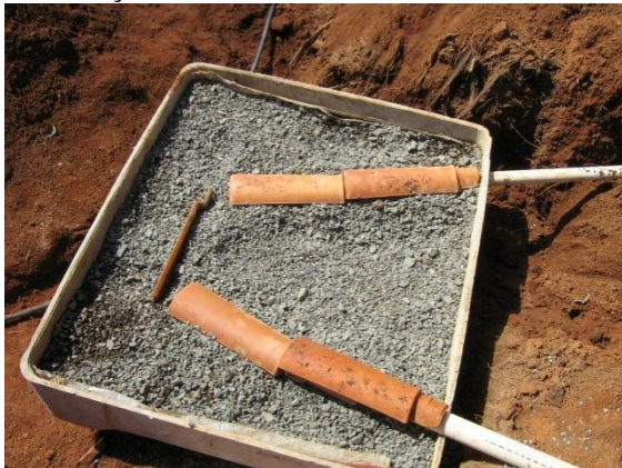
(c) preenchimento com pedra brita no. 1.
