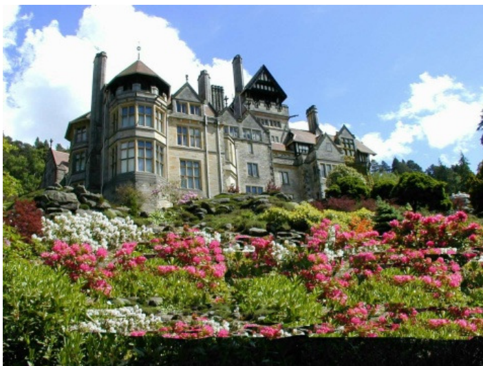
FIGURA 4 - Cragside House (fonte: CRAGSIDE, 2007)
