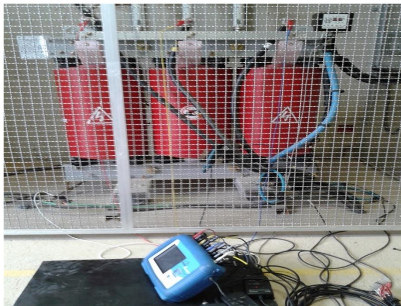
Figure 7.4– PQ Analyser installed at the output of the distribution transformer in the building (OLIVEIRA et al., 2015).
