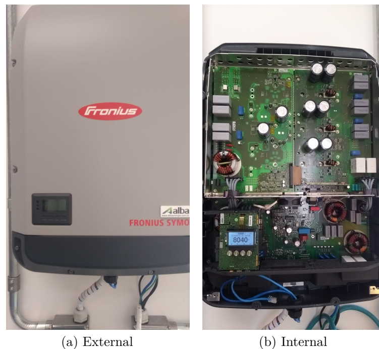
Figure 39 – Fronius Symo 12.5 3M Inverter.
