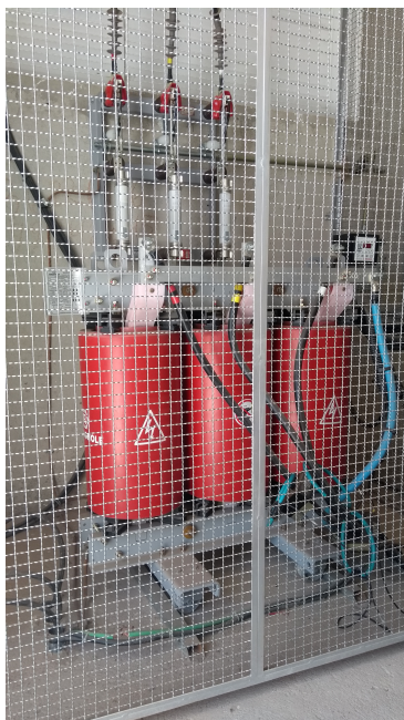
Figure 37 – Medium Voltage Transformer.
