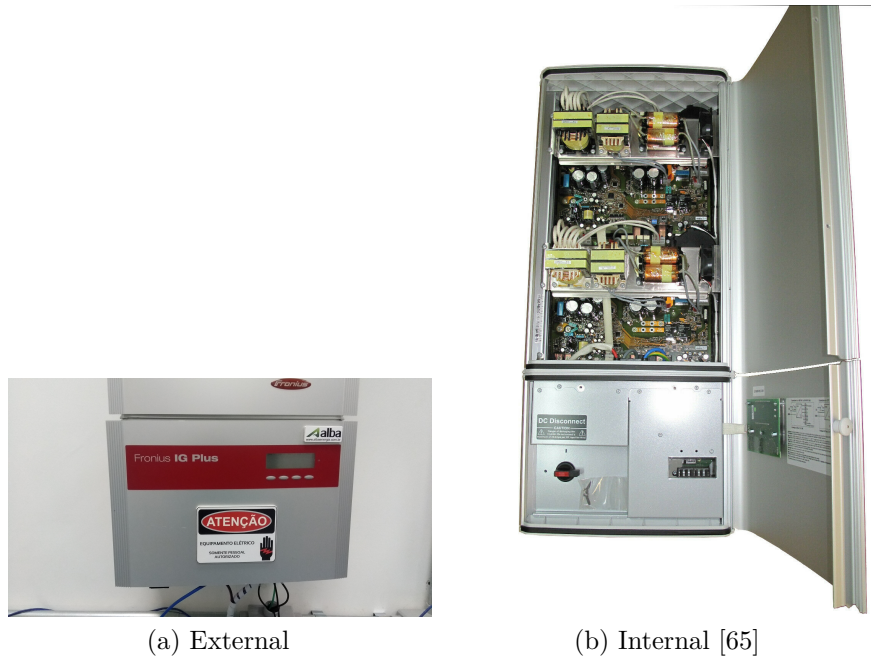
Figure 40 – Fronius IG Plus 100 V-3 Inverter.
