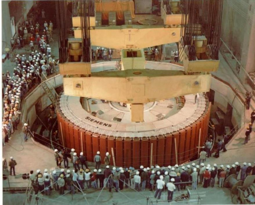
Figure 2.5 –SG salient poles rotor being installed in Itaipu, 1760 ton, and 90 rpm.
