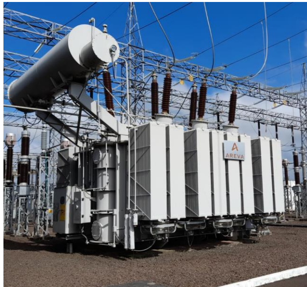
Figura 5 - Resfriamento Oil Natural Air Forced (ONAF)
