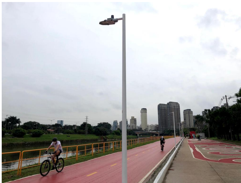
Figure 21 – Street Light Solution.
