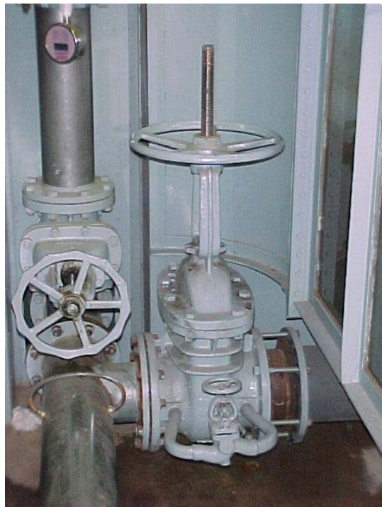
Figura III.13 – Válvula gaveta
