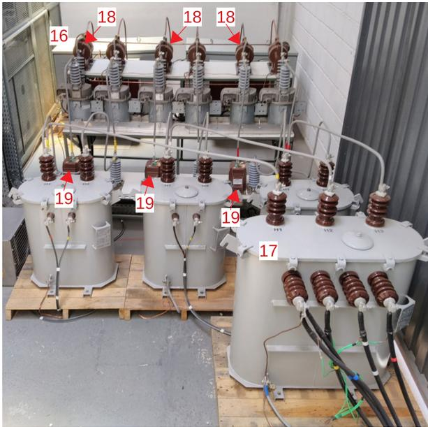
FIGURE 18. Test 13.8 kV substation.
