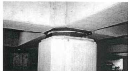
Hayward City Hall Installed Bearing
