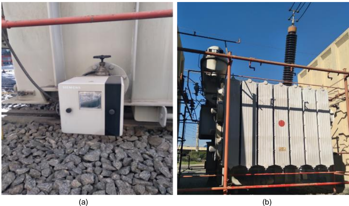
Figure 6.1 – Real case of (a) continuous online oil monitoring system installed on a (b) power transformer in operation, installed in an ISA CTEEP substation.
