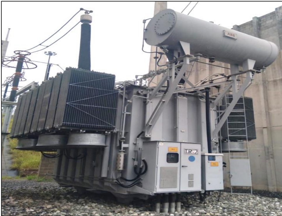
Figure 1.1 – Power transformer in operation, installed in an ISA CTEEP substation [5].
