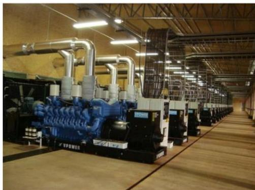
Figure 8. Part of the 99 generating units of the Palmeiras de Goiás Thermal Power Plant.
