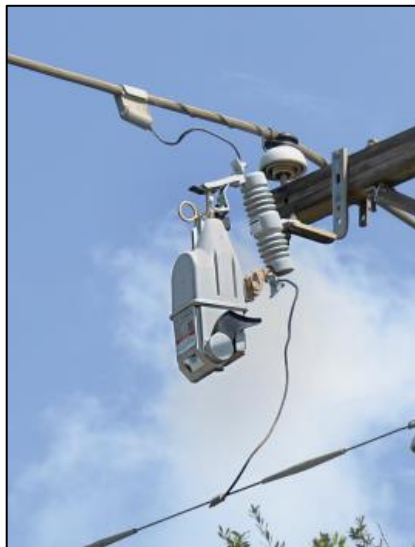
Figura 2.19 – TripSaver (S&C, 2020)
