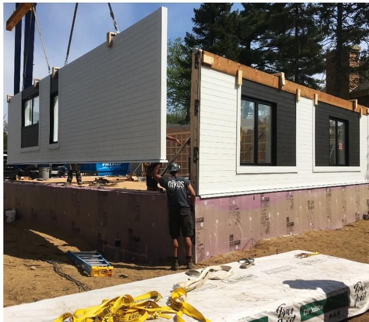
**Figure 11.** Picture taken during the installation of the studied wall.
